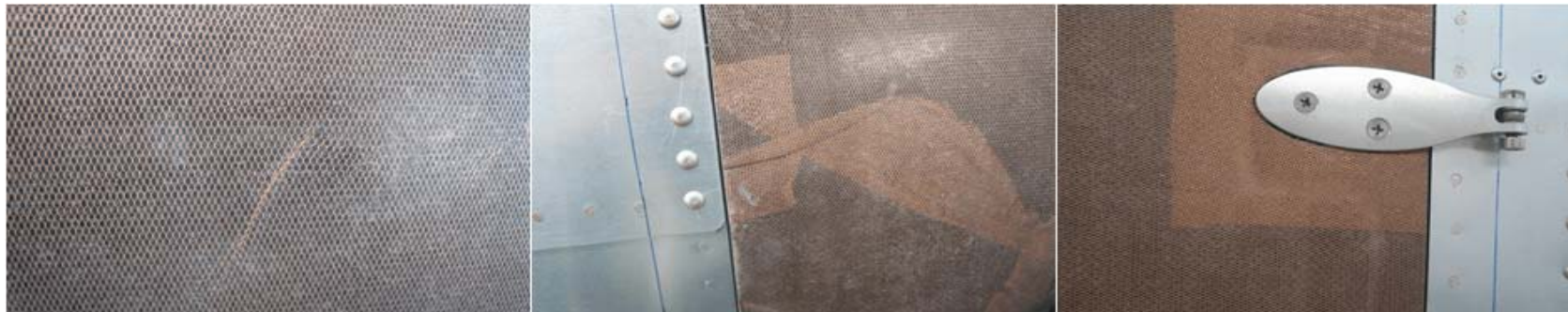
Materials defects on protected composite
