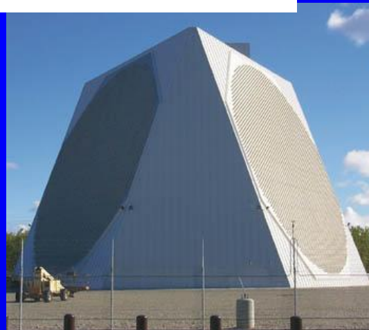
Courtesy of Alaska District, this 90-foot (27m) diameter radar installation monitors the northern sky. Its construction was part of the Clear Radar Upgrade to make all Ballistic Missile Early Warning System radars phased-array rather than mechanical.
